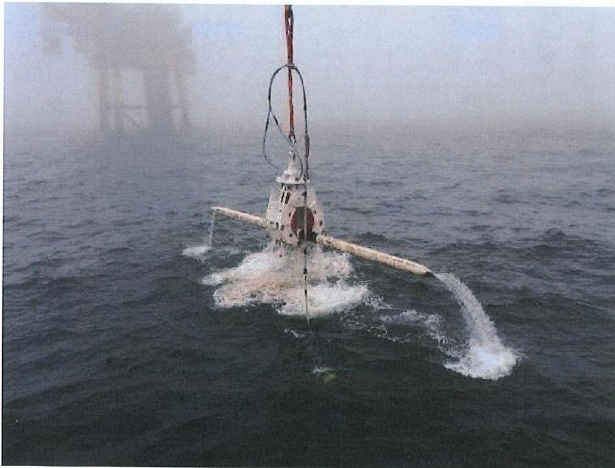
Figure 5 Recovering Cut Pipe section with Hydraulic Grapple
